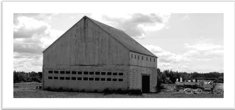
This 1863 image shows the (fake) train wheel replacement barn above Plant One during the Civil War. The 12’ walls around Camp Chase sat about a thousand feet beyond those background trees.
